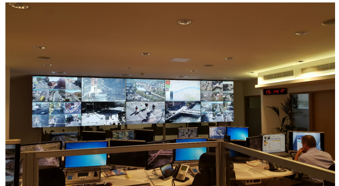
Figure 1: The traffic control room at Dublin City Council, where different monitors visualize the traffic conditions at different locations in the city of Dublin, captured from CCTV cameras, and allow traffic operators to monitor the traffic conditions
